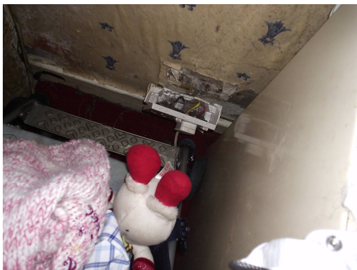
Picture 3 showing a Broken Electrical Plug Socket.
